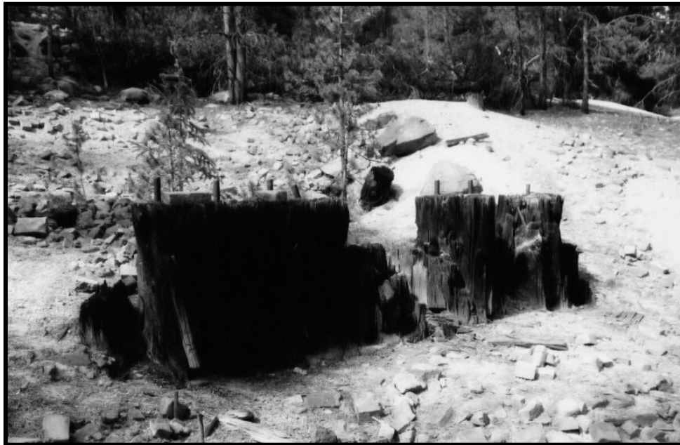
Illustration A 1.4.50: When a stamp battery was dismantled, the pedestals for the cast iron battery boxes were often left in place. The pedestals consist of timbers on-end and feature anchor bolts on top, and each is around 2' wide, 3' high, and 5' long. Source: Eric Twitty, 2009.
