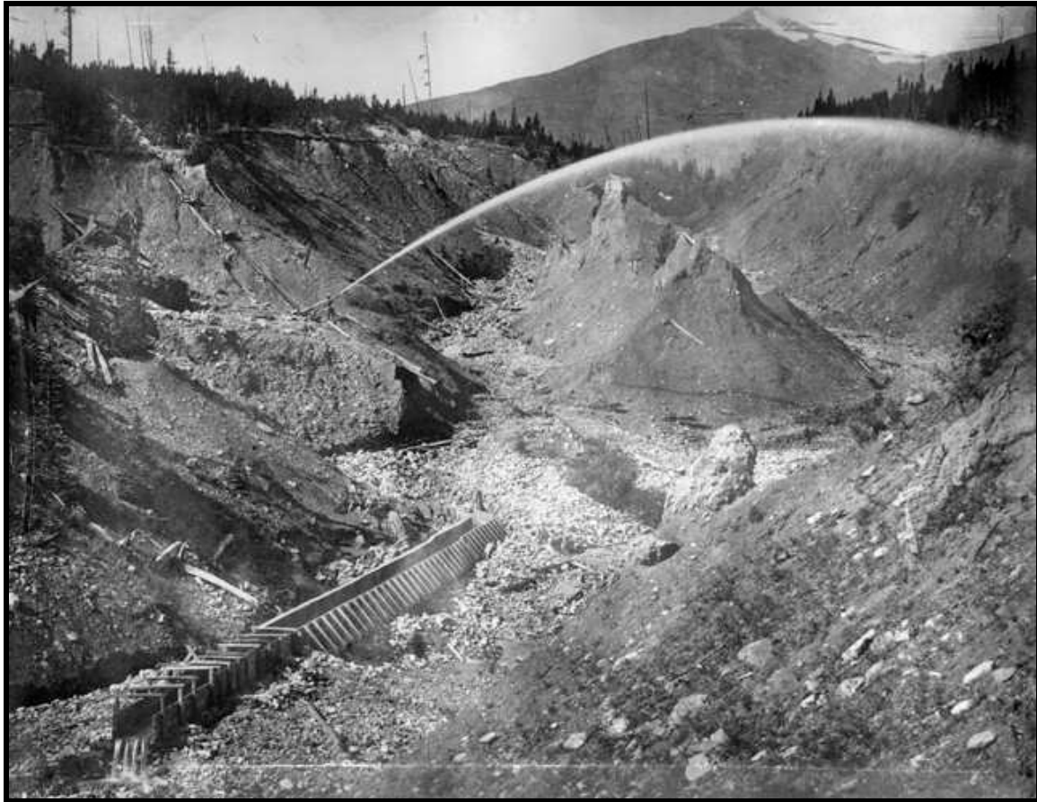
Illustration B 1.4: Hydraulic mines followed a common pattern in engineering and workings. Monitors emitted high-pressure jets of water that eroded gold-bearing gravel and washed slurry through a system of sluices. The operation in the photo was the Iowa Hill Mine near Breckenridge, Summit County, during the 1880s. Courtesy of Breckenridge town historian Rebecca Waugh.
