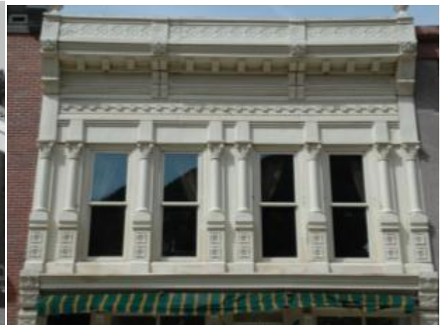
Illustration B 8.17: Mahr Building, Telluride, Colorado, with 1892 Mesker Bros. cast iron facade. Source: Carl McWilliams, 2007.
