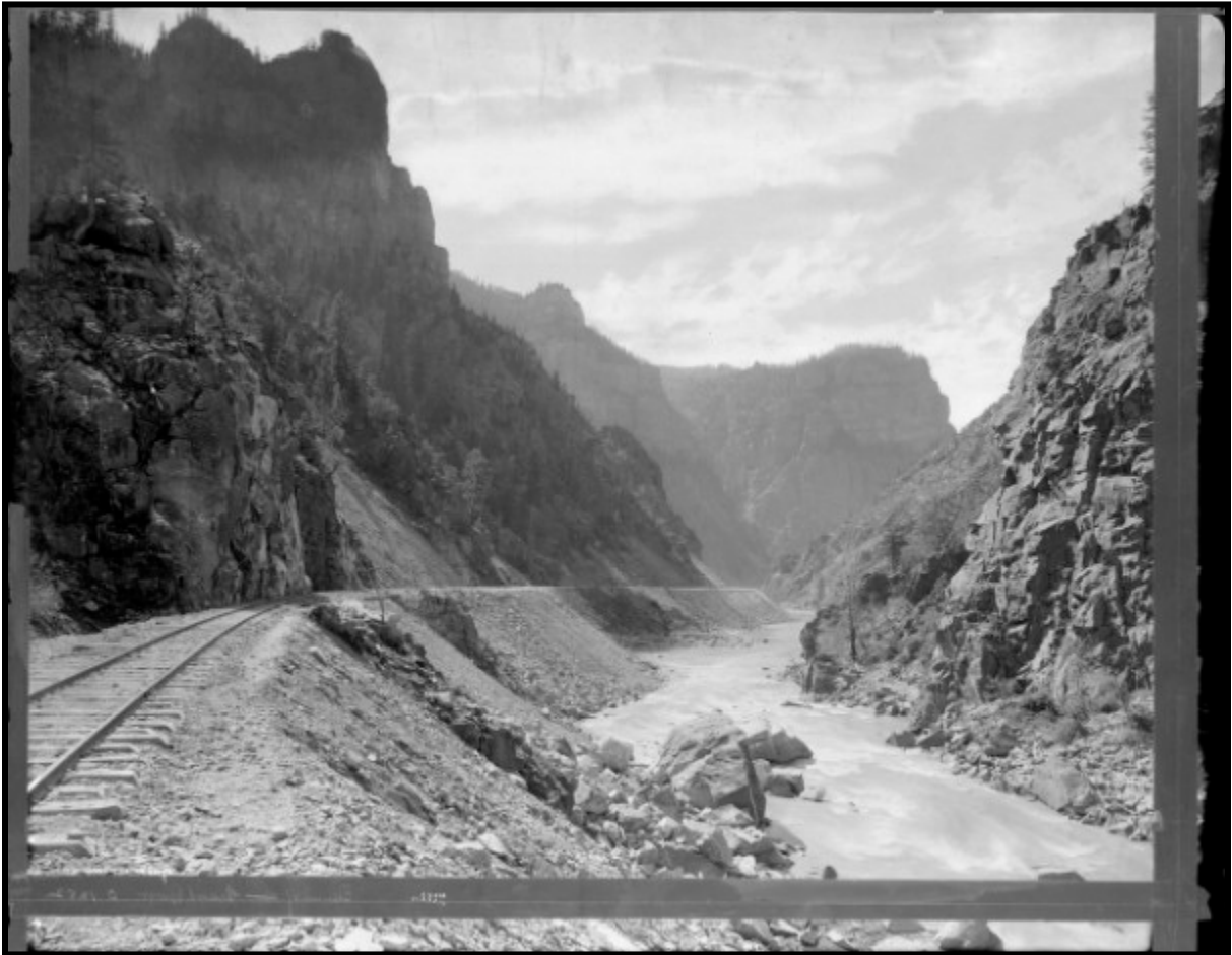
Illustration B 5.1: The late 1880s William Henry Jackson photo of the Denver & Rio Grande line through Glenwood Canyon exemplifies a typical railroad grade and common characteristics. Evident are cuts and fills to level the grade, and gentle curves and straight lines required by locomotives. The track consists of rails, ties, and a veneer of ballast over the carefully flattened surface of the gravel bed. Courtesy of Denver Public Library, CHS.J3885.
