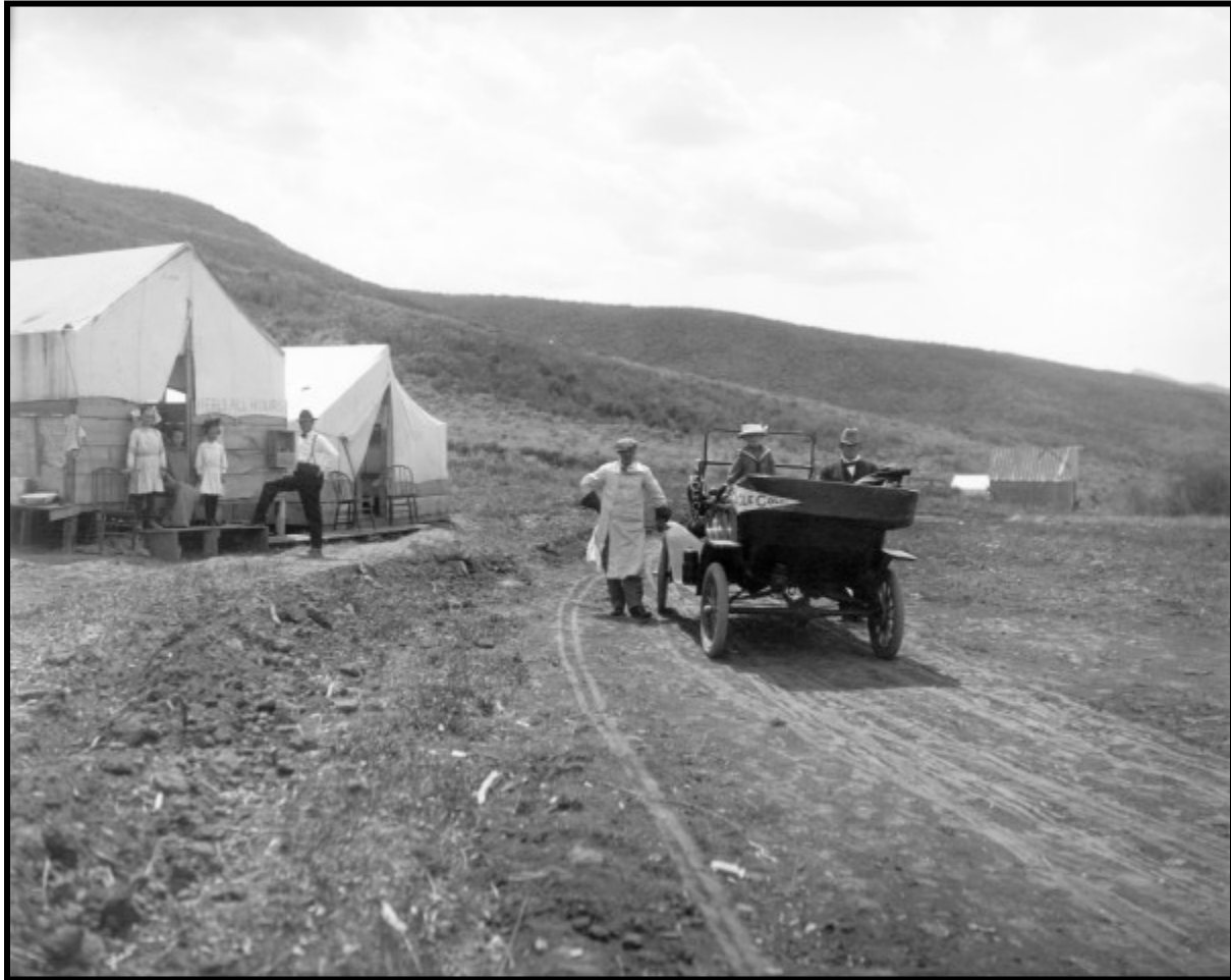
Illustration B 1.16: The prospector's camp photographed on Horse Mountain south of Eagle in 1913 reflects how field accommodations changed little since the 1860s. The camp is typical with several wall tents on a cut-and-fill platform, and few if any other improvements. Courtesy of Denver Public Library, CHS-X5655.
