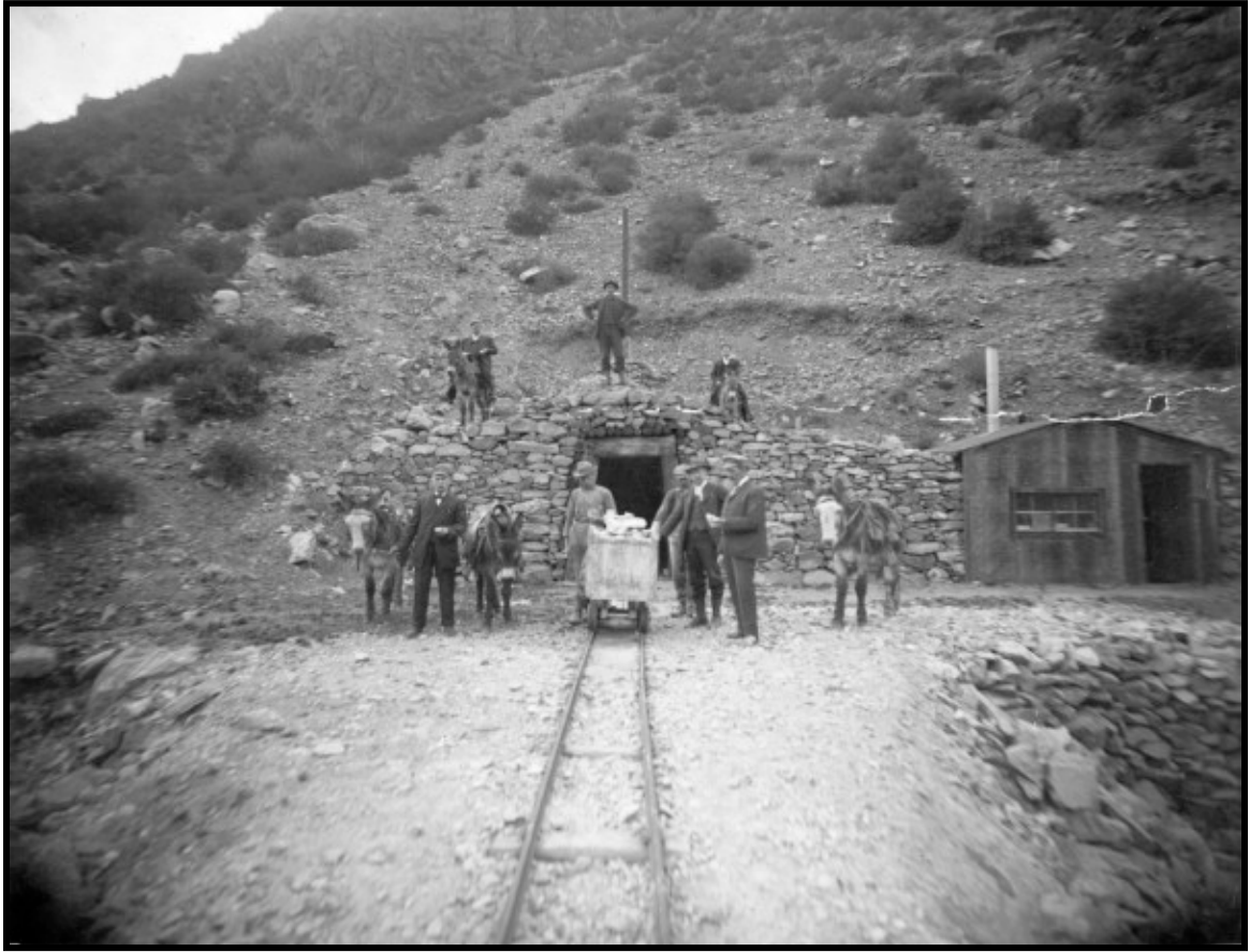
Illustration B 1.7: Most tunnel mines, such as this operation near Georgetown during the 1890s, were small and simple. Surface facilities consisted of a blacksmith shop, tunnel portal, rail line, ore bin, and little else. Even when buildings and structures are gone, tunnel mines may be eligible for the NRHP if the archaeological features and artifacts clearly represent the operation. Courtesy of Denver Public Library, X-61651.
