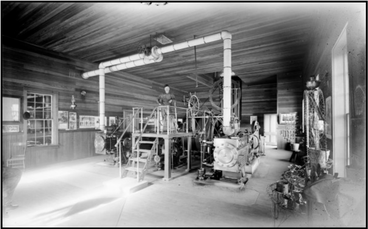
Illustration A 1.4.20: The rear quarterview illustrates a first-motion, double-drum hoist at the Gehrman Shaft, Stanley Mine, west of Idaho Springs around 1900. The hoist operator relied on the circular level gauge above the large machine to determine where in the shaft the cage vehicles were, exactly. The hoist room is immaculate, maps line the walls, and potted plants are by the window at right. Courtesy of Denver Public Library, CHS-B337.
