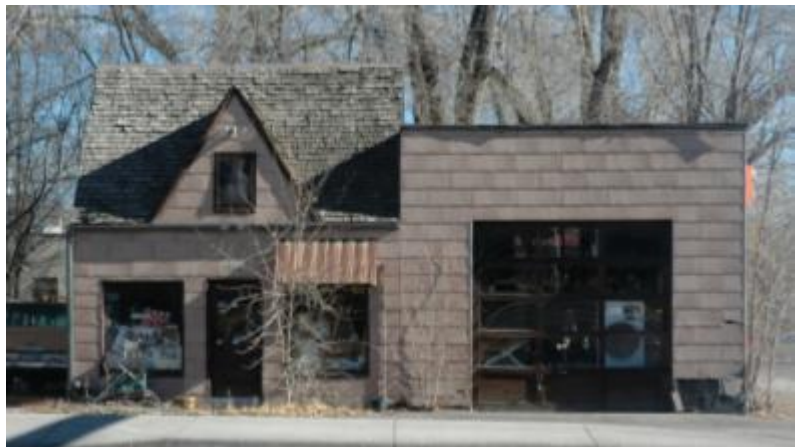
Illustration B 8.22: Cottage filling station with attached service bay, Longmont, Colorado. Source: Carl McWilliams, 2010
