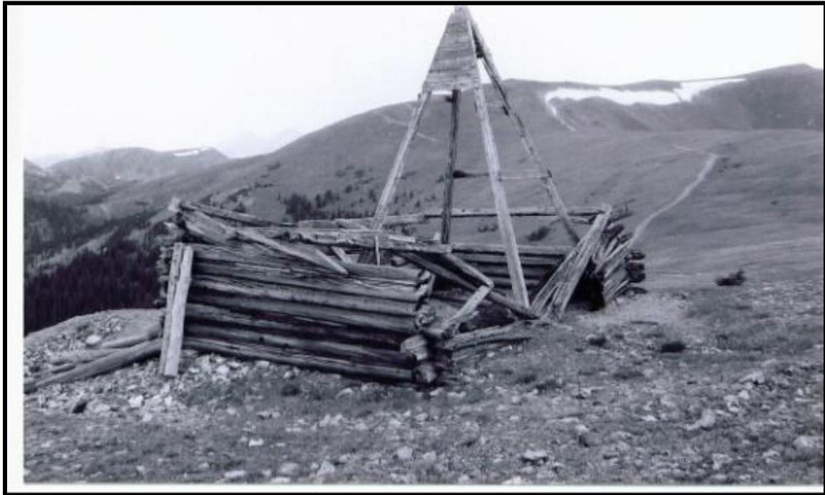
Illustration B 1.5: The Thompson Mine near Breckenridge in 2003, is characteristic of deep prospect shafts. These operations typically had a simple headframe and blacksmith shop enclosed in a shaft house. Additional property development is absent, and the waste rock dump limited in volume. Archaeological features represent the buildings and structures at most sites. Source: Eric Twitty.
