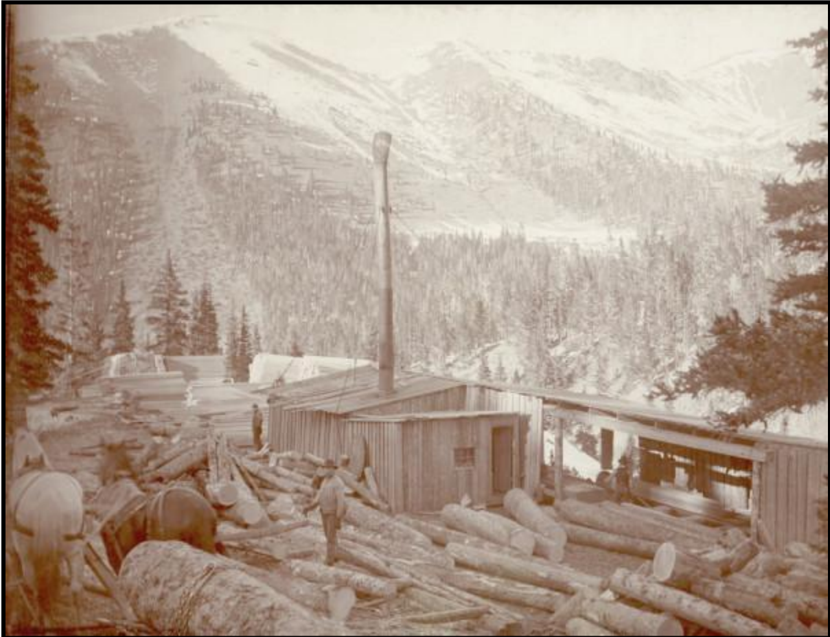
Illustration A 2.1: The Wapiti Sawmill typifies most lumber facilities in the I-70 Mountain Corridor. Workers rolled logs from a stockpile in the foreground onto a dolly in the mill, before feeding them into saw-blades. The dolly is at right, and the saw-blades, steam engine, and boiler are in the building at center. The mill, in this northerly view, operated between Breckenridge and Dillon for the Victoria Mining Company around 1890. Courtesy of Denver Public Library, X4929.
