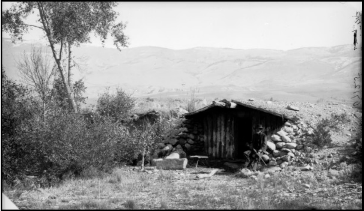
Illustration A 3.1: This bunker-like structure in the Colorado River valley, photographed during the 1880s, is a typical homesteader's dugout. Its primitive façade and lack of windows indicate that it was temporary, later to be replaced by a cabin or house. Courtesy of Denver Public Library, CHS.J959.
