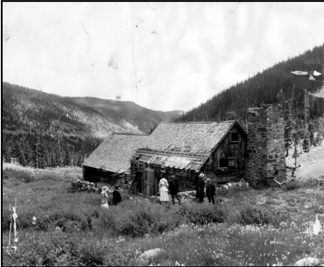
Illustration B 1.15: When the Dibben Smelter at Argentine was photographed during the late 1890s, it had already been long abandoned. The facility is typical of the smelters built in Clear Creek drainage during the late 1860s and early 1870s, with local stone chimney and furnace, and small building built over several stairstep foundations. Masonry and foundations are all that remain from most smelters of the vintage. Courtesy of Denver Public Library, X-61397.
