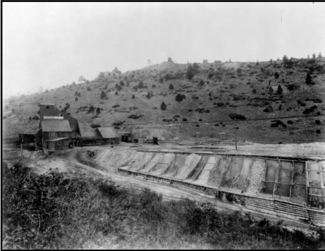
Illustration B 1.6: The Gem Mine on Seaton Mountain above Idaho Springs around 1910 typifies large, professionally engineered shaft operations. A complex shaft house enclosing the shaft collar, hoisting system, steam boilers, and shop stands at left. A large waste rock dump and series of ore bins extends right. Most mines were not as extensive as the Gem but featured similar characteristics. Courtesy of Denver Public Library, X-60758.
