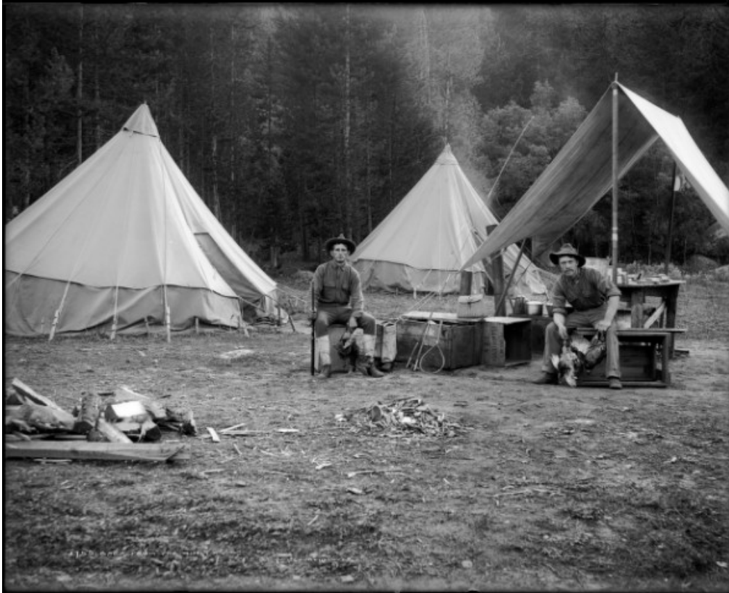
Illustration B 7.1: Photographed by Charles McClure between 1900 and 1920, this hunting camp near Norris is typical of the era, with several tents, table under a shelter, and sheet iron stove. Fishing camps were similar. Courtesy of Denver Public Library, MCC-1755.
