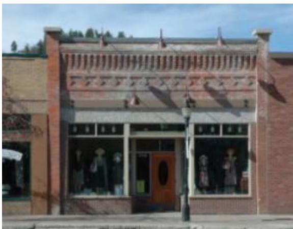
Illustration B 8.20: Skee Inn Cafe, Early Twentieth Century Commercial building, Steamboat Springs, Colorado. Source: Carl McWilliams, 2007.
