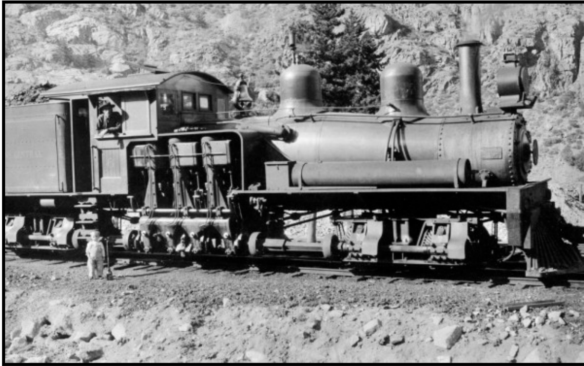
Illustration A 5.8: This side-gear locomotive, known as a Shay design, made the Argentine Central Railroad possible. The Shay was the only type capable of pulling cars up the tortuous and steep grades from Silver Plume into the Argentine Mining District. The photo was taken on the Argentine Central around 1910. Courtesy of Denver Public Library, X-17687.
