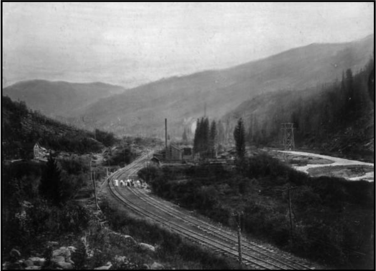
Illustration A 5.13: The Colorado & Southern Railroad assumed the High Line from Dillon to Leadville in 1898 and continued service through Summit County. The route was instrumental in the region's late 1890s mining boom. The southwest view up Ten Mile Canyon, by Otto Westerman around 1908, shows the Mary Verna Powerhouse and siding at Curtin. I-70 was graded later on the canyon's far right side. Courtesy of Denver Public Library, X-62731.
