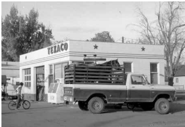
Illustration B 8.24: Texaco Oblong Box filling station, Ignacio, Colorado. Courtesy Denver Public Library, X-17788, ca. 1980-1990
