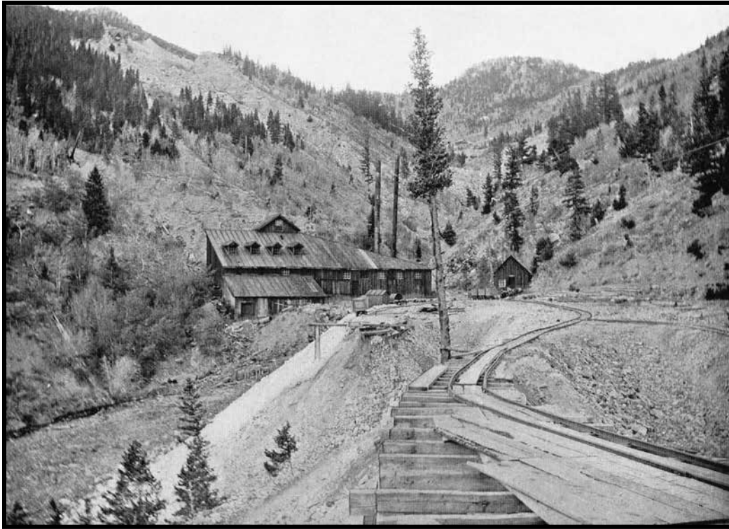
Illustration A 1.2.24: The Aorta Tunnel was among Empire's earliest profitable mines but went idle during the 1880s. During the late 1890s, the Empress Mining & Tunnel Company lengthened the tunnel as a deep haulage way for other mines. The operation became one of Empire's most important. The mill, a good example of an amalgamation stamp mill, may have been built by the Bay State Mining Company during the 1860s. Photo date is uncertain, although likely in the 1890s. Source: Spurr, 1908.
