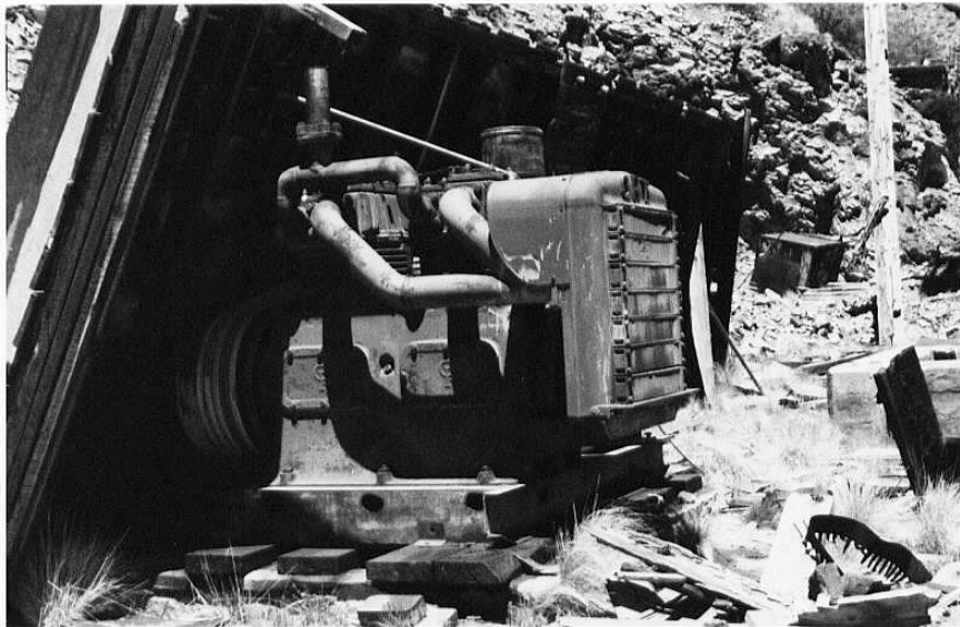
Illustration A 1.4.38: The V-cylinder compressor, similar to a large engine, became one of the most popular compressor types during the 1930s. Note the foundation. Source: Eric Twitty, 1999.
