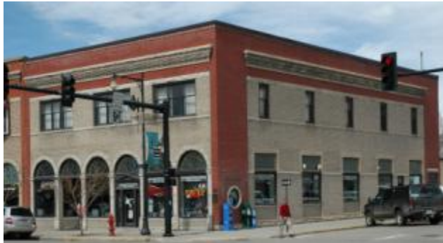
Illustration B 8.19: Routt County National Bank, Early Twentieth Century Commercial building, Steamboat Springs, Colorado. Source: Carl McWilliams, 2007.
