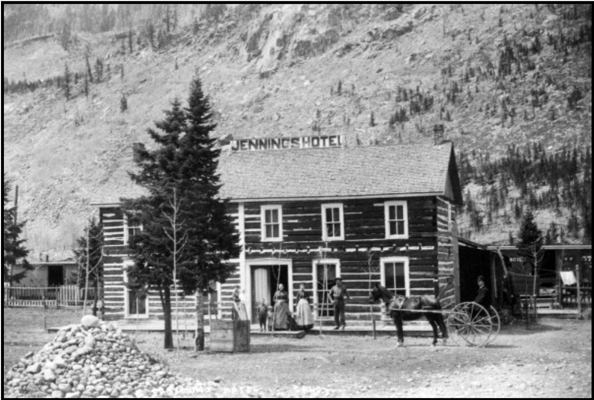
Illustration A 7.4: Mountaineers, few in number during the nineteenth century, stayed in the Jennings Hotel at Graymont before and after testing themselves against Gray's and Torrey's peaks. The hotel, photographed by George Dagleish around 1884, gave the mountaineers a taste of frontier accommodations until the railroad ended service in 1893. Courtesy of Denver Public Library, X-8760.
