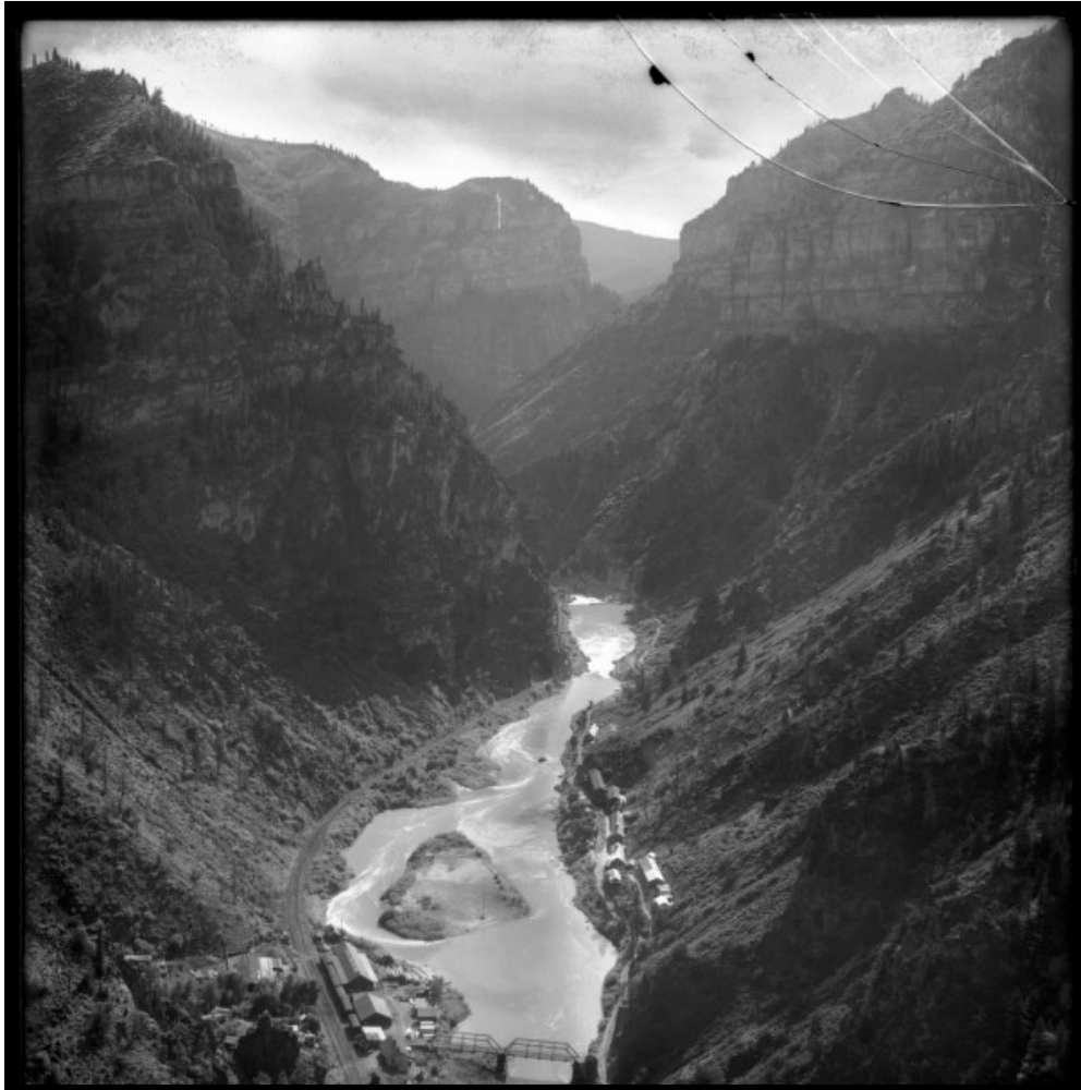
Illustration A 4.9: In 1906, the Central Colorado Power Company erected the settlement of Shoshone on the left (south) side of the Colorado River to house workers building a massive hydro-plant on the right side. The camp was no longer needed after they finished in 1911, so the company dismantled it. Courtesy of Denver Public Library, MCC.3804.
