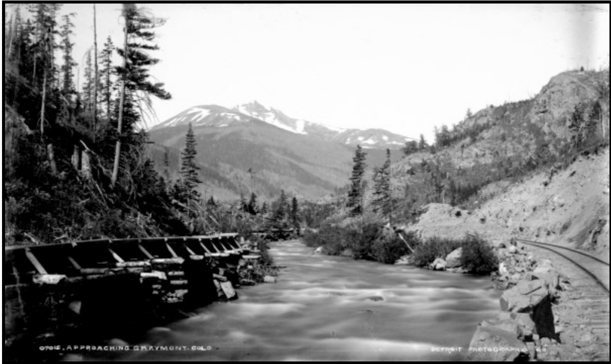
Illustration A 2.5: The Clear Creek Flume, left, and Georgetown, Breckenridge & Leadville Railroad, right, granted lumber companies in upper Clear Creek drainage two means of shipping forest products to market. As a result, lumber companies quickly exhausted the forests, evident by the large clear cuts in the background of this 1885 photo of the Bakerville area. Courtesy of Denver Public Library, CHS-J882.
