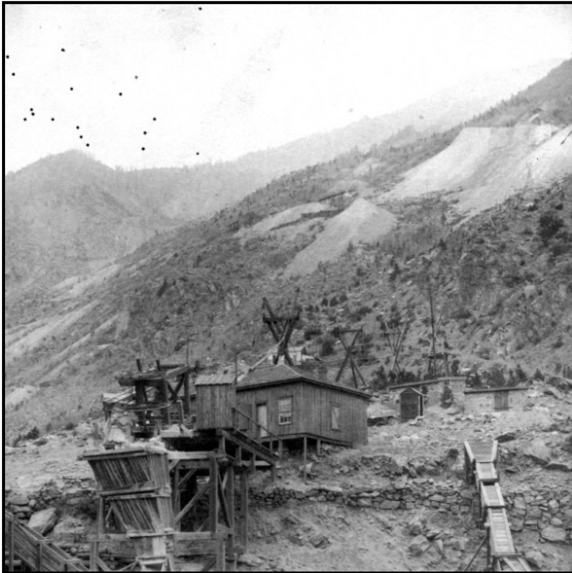
Illustration A 1.4.44: At the Pay Rock Mine near Silver Plume, a Hallidie tramway lowered ore from workings high on the mountainside down to a bottom terminal and loading station. The sheave wheel is enclosed in the slanted frame above the ore bin. The towers are unusual tripod structures. Courtesy of Denver Public Library, CHS.X4578.
