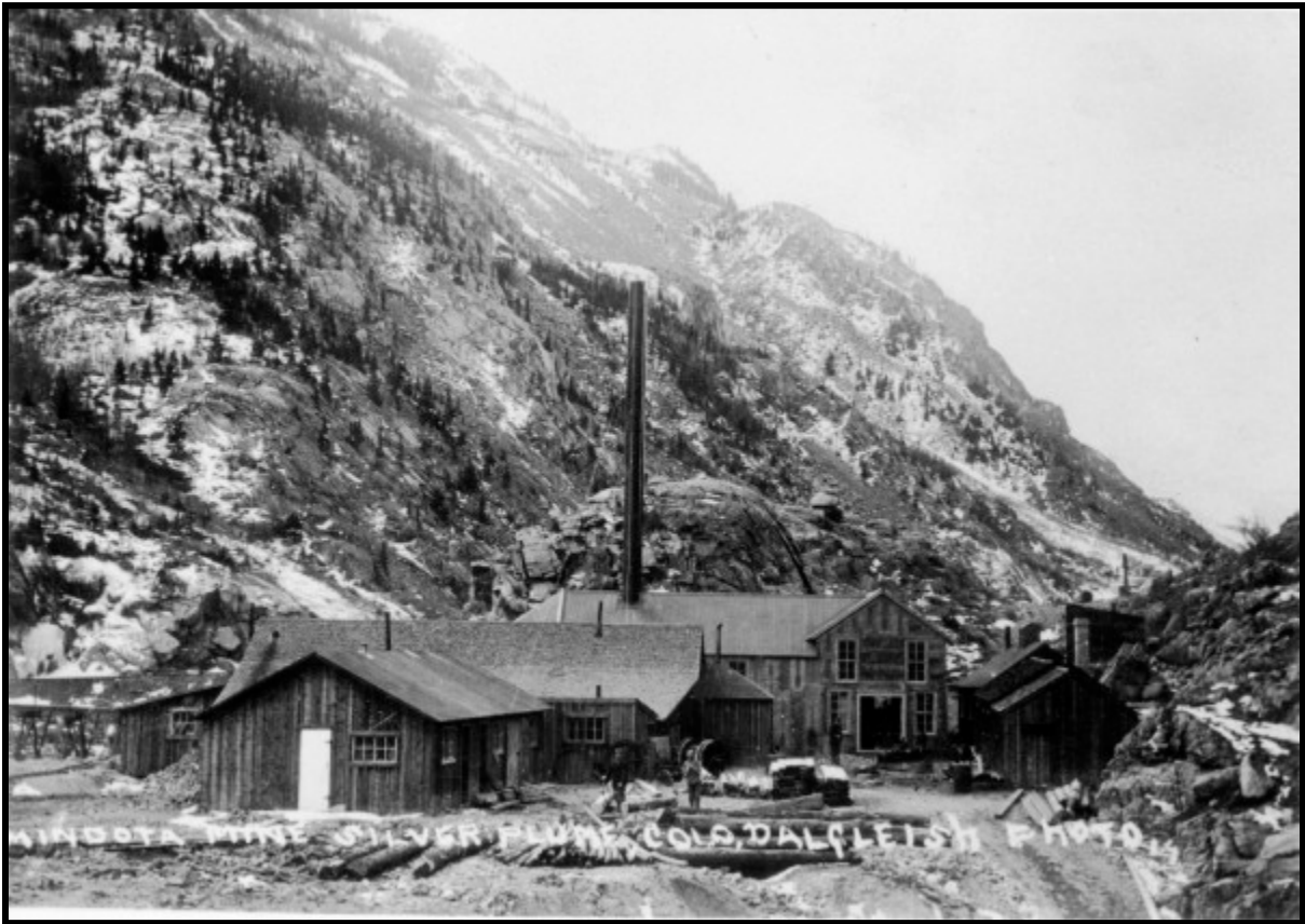
Illustration A1.4.40: The buildings at the Mendota Mine, Silver Plume, are typical of professionally designed, vernacular architecture specific to the mining industry. The building with smokestack is a tunnel house enclosing a blacksmith shop, air compressor and boiler, and tunnel portal. The other buildings are an office and more shop space. The buildings were probably custom-designed by a company official for function and economy, rather than appearance. Board-and-batten siding and shingle roofing was common into the 1910s, when corrugated sheet iron became universal. Courtesy of Denver Public Library, X-61693.
