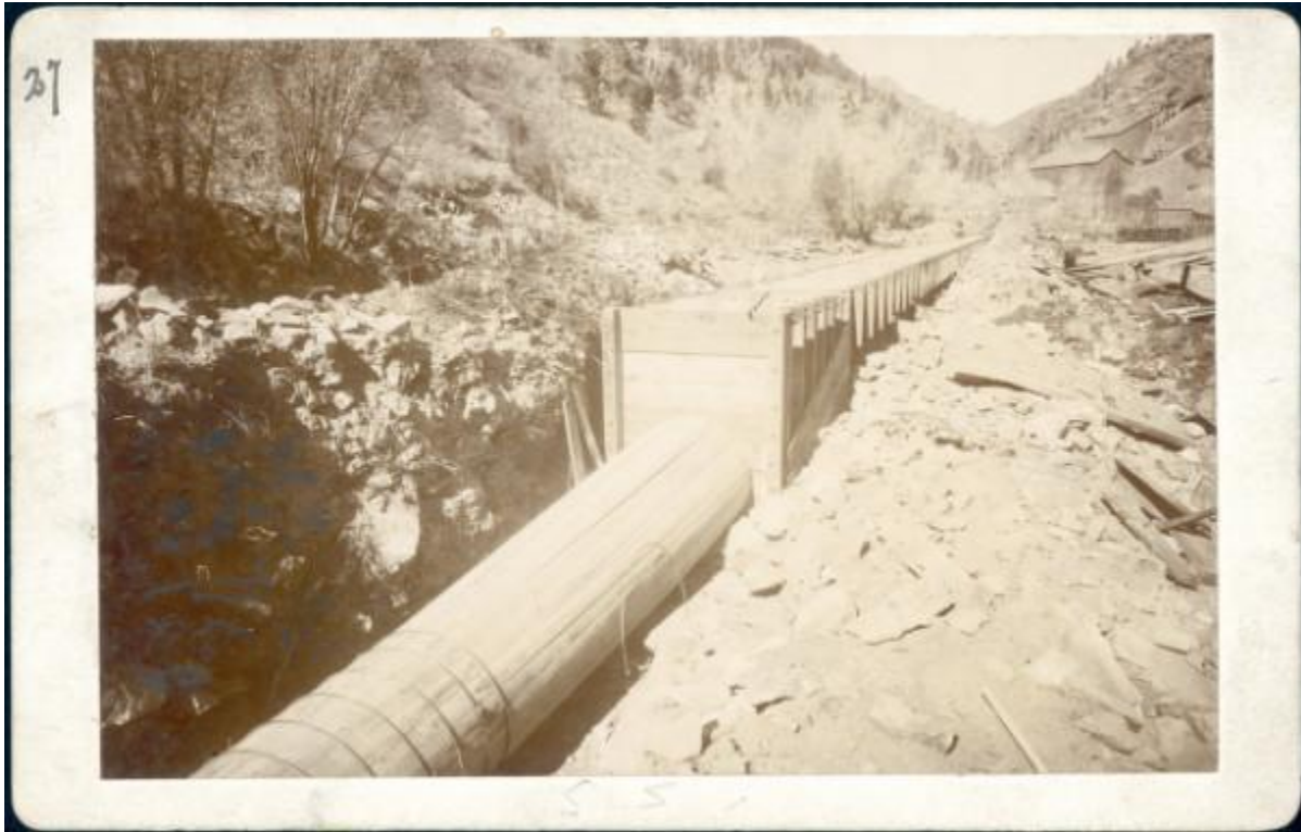
Illustration B 4.4: Infrastructure components include facilities and constructs in support of powerplants and their electric grids. Flumes and pipelines for hydropower, such as these in construction for the Stanley Mine near Idaho Springs in 1894, are the most common. Many have been dismantled and are now represented by archaeological features. Lachlan McLean took the photo. Courtesy of Denver Public Library, Z-4767.
