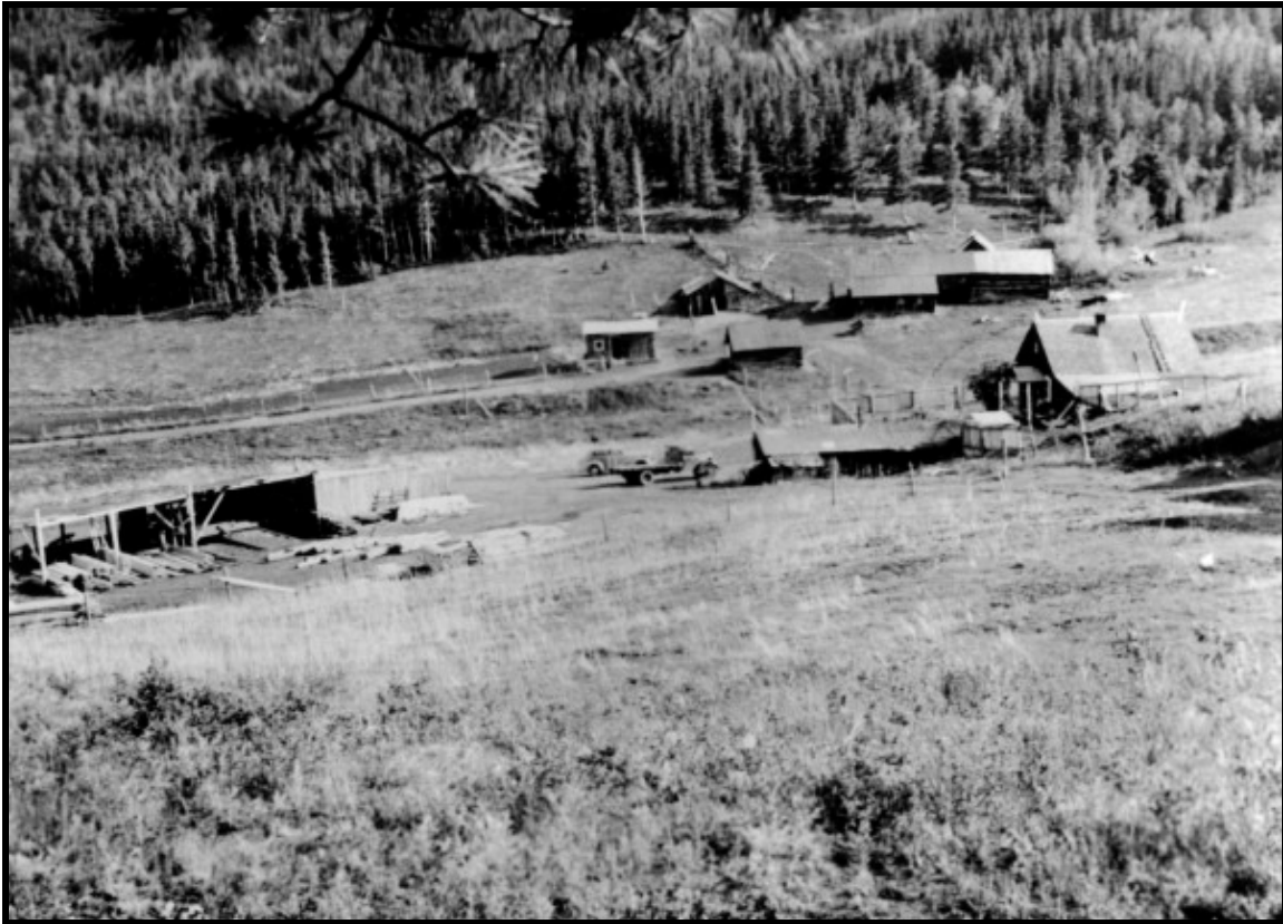
Illustration B 2.1: Most of the sawmills in the I-70 corridor were small facilities such as this one photographed near Silver Plume in 1938. They were simple for portability and relocation to fresh forests. The sawmill, frame enclosing the saw-frame, and building surrounding the saw-blades and engine are at left. Finished lumber and logs are stockpiled near center, and workers' housing is right. Courtesy of Denver Public Library, X-17668.
