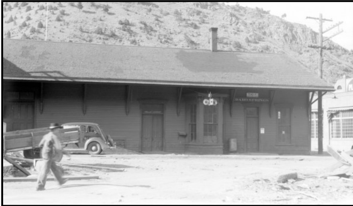
Illustration B 5.3: The Idaho Springs railroad depot, depicted by Otto Perry in 1941, was a combination type with typical architectural characteristics, including bay window, service doors, and deep roof overhang. The railroad tracks are on the other side. Courtesy of Denver Public Library, OP-6385.
