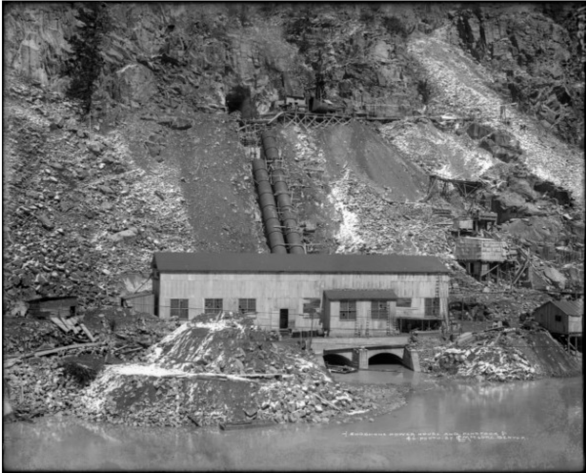
Illustration A 4.11: The Shoshone powerhouse, under construction in this Charles McClure 1908 photo, became the western terminus of a grid linking most of the principal towns in the central mountains. Water diverted from a dam upriver flowed through the tunnel in the cliff above, down through the penstocks, and into the building. Although modified, the system is still in operation today. Courtesy of Denver Public Library, MCC-3397.
