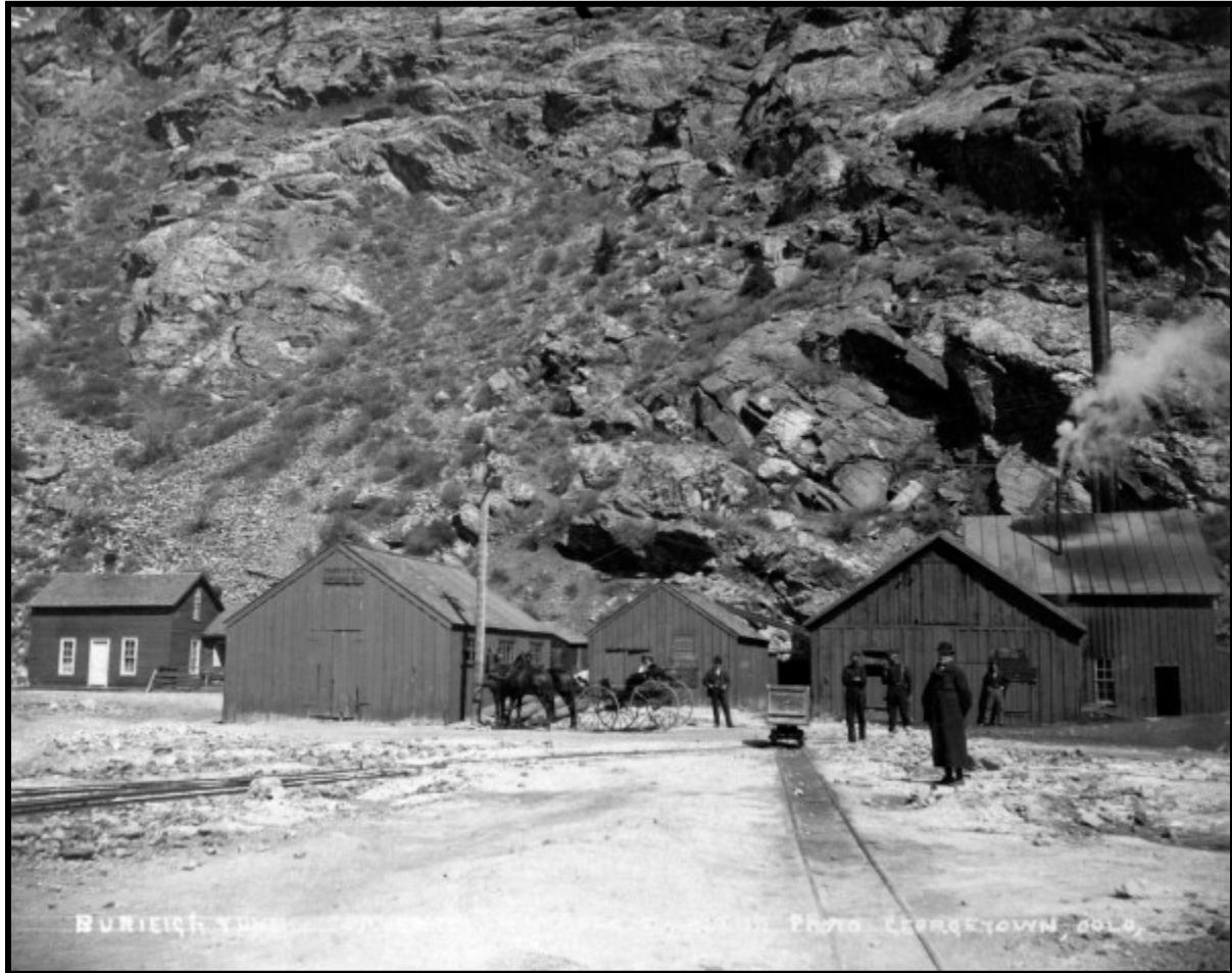
Illustration A 1.2.10: The Burleigh Tunnel was among the most important operations in western Clear Creek drainage during the late 1860s and early 1870s. Not only was the tunnel a major capital investment, but also proved that the ore veins around Silver Plume held value at depth, which many investors began to question at the time. Further, Charles Burleigh pioneered the use of rockdrills for drilling blast-holes underground, which revolutionized the greater mining industry in later decades. George Dalgleish took this north view during the 1880s. Courtesy of Denver Public Library, X-61687.
