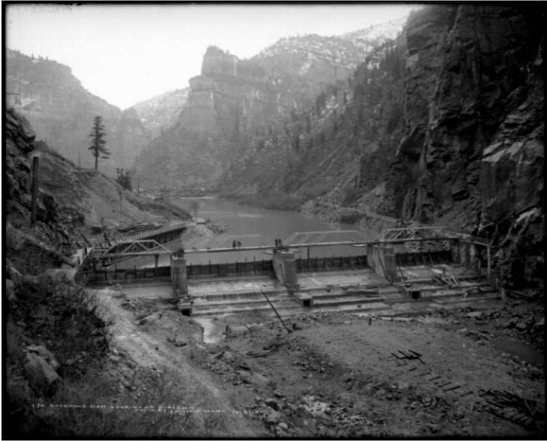
Illustration A 4.10: The Shoshone Dam, on the Colorado River several miles above the powerhouse, was an engineering achievement. Steel gates known as bear traps could be raised or lowered, depending on river flow, to ensure diversion into the powerplant's intake tunnel in the cliff at the left side. Charles McClure captured the upstream view in 1910. Courtesy of Denver Public Library, MCC-3850.
