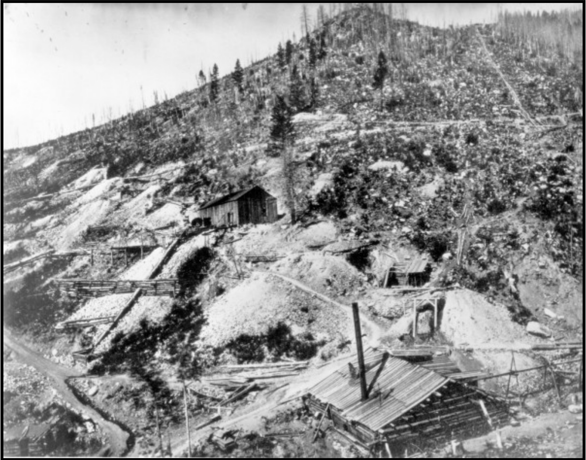
Illustration B 1.9: Some mines, such as the Tenth Legion near Empire during the late 1860s, were a complex series of workings on a linear ore vein. In the photo, miners developed the upper portion through a shaft, marked by a shaft house at center, and the lower portion through a tunnel, with a log shop building at the lower right. Open-cuts exposed the vein in between. Note the ore chutes and log cribbing walls retaining waste rock. Courtesy of Denver Public Library, X-61589.
