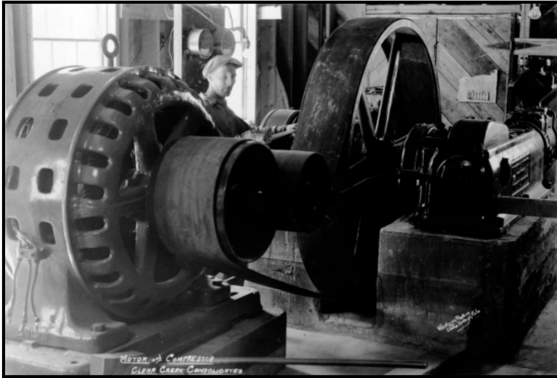
Illustration A 4.3: Mining companies gradually replaced old steam equipment with motorized versions, such as this belt-driven air compressor at the Clear Creek Consolidated operation near Idaho Springs around 1900. Motors saved companies the costs of installing boilers and feeding them coal. Courtesy of Denver Public Library, X-63213.
